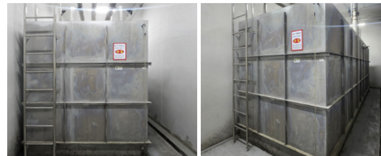
<Water Resource Facilities>
